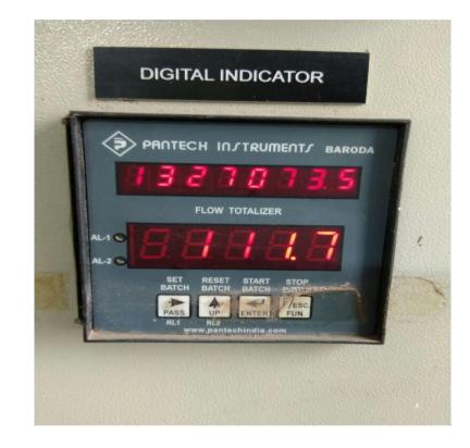
Flow totalizer provided on Nylon-6 II DCS of flow meter installed on Nylon-6 II effluent line to ETP
